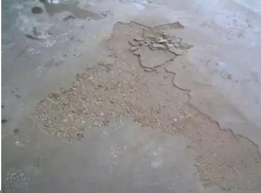
Fig 4: Delamination
