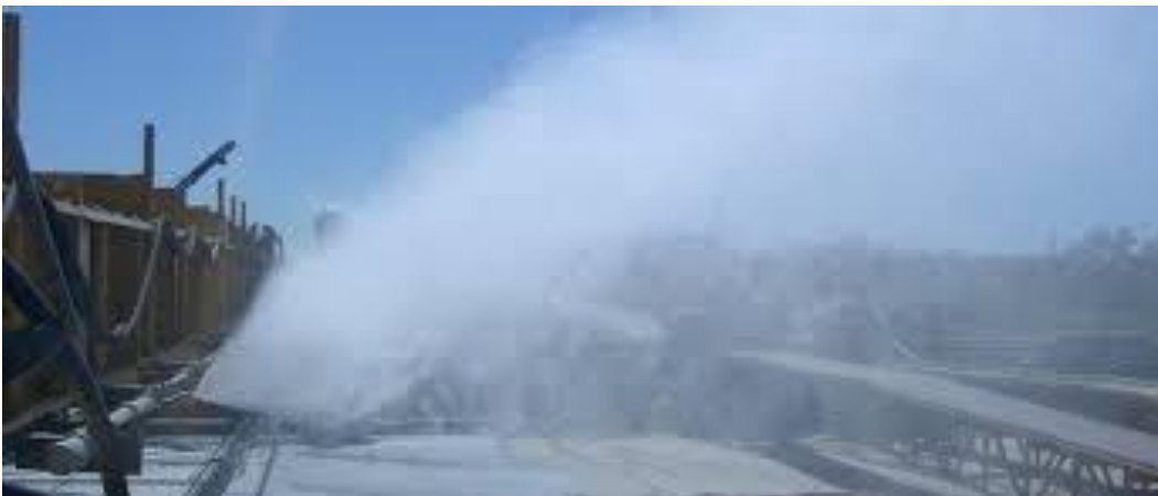
Fig.: Steam curing of concrete
