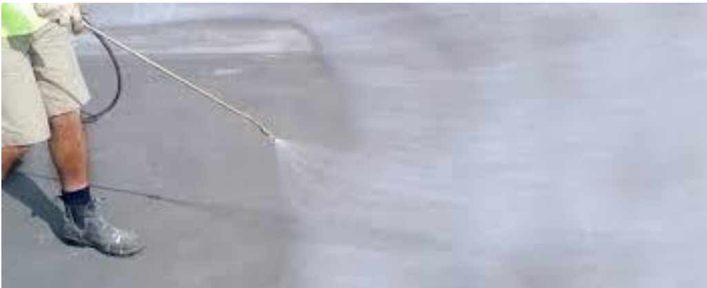
Fig.: Curing by the sprinkling of water
