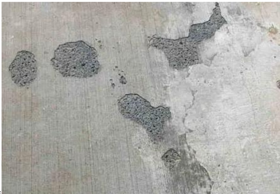
Fig 3: Concrete Blisters
