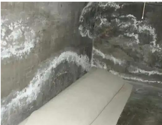
Fig 7: Efflorescence
